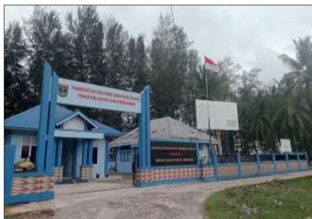
5. INSTALASI KKD BATANG GASAN
